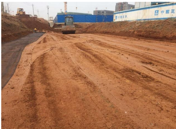
纵一路清表及路基筑填 (2017. 3. 7)
